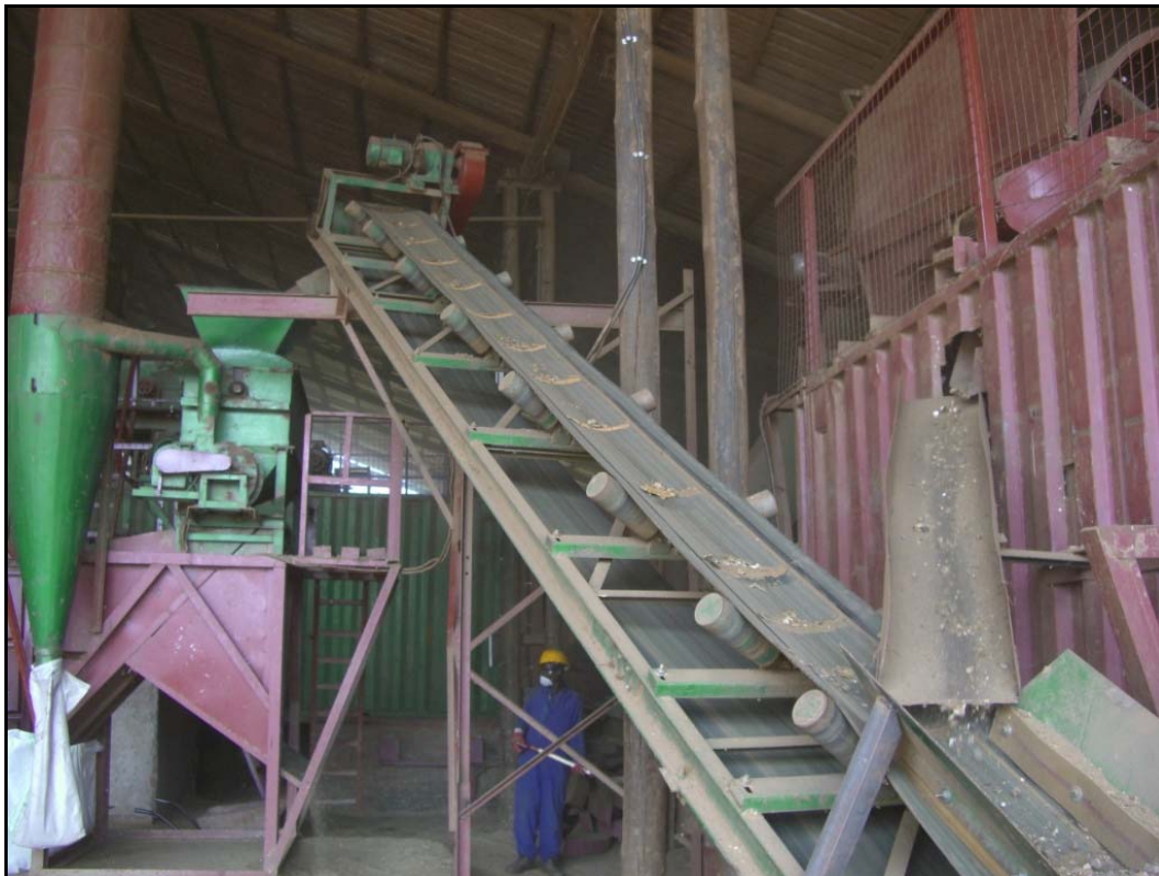
Namekara Plant Operational
